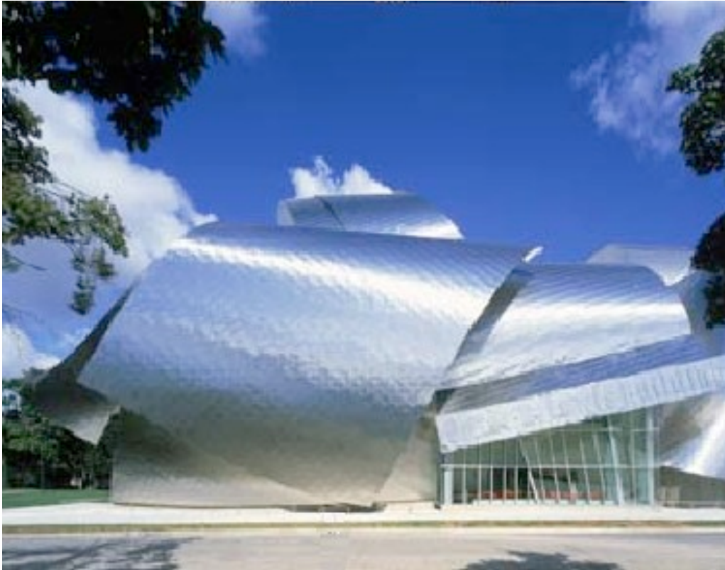
REGIONAL AUTOMATED MANUFACTURING TECHNOLOGY AND EDUCATION CENTER
